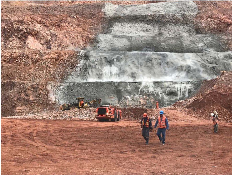
Figure 3: Portal Location Prior to Commencement of Development
