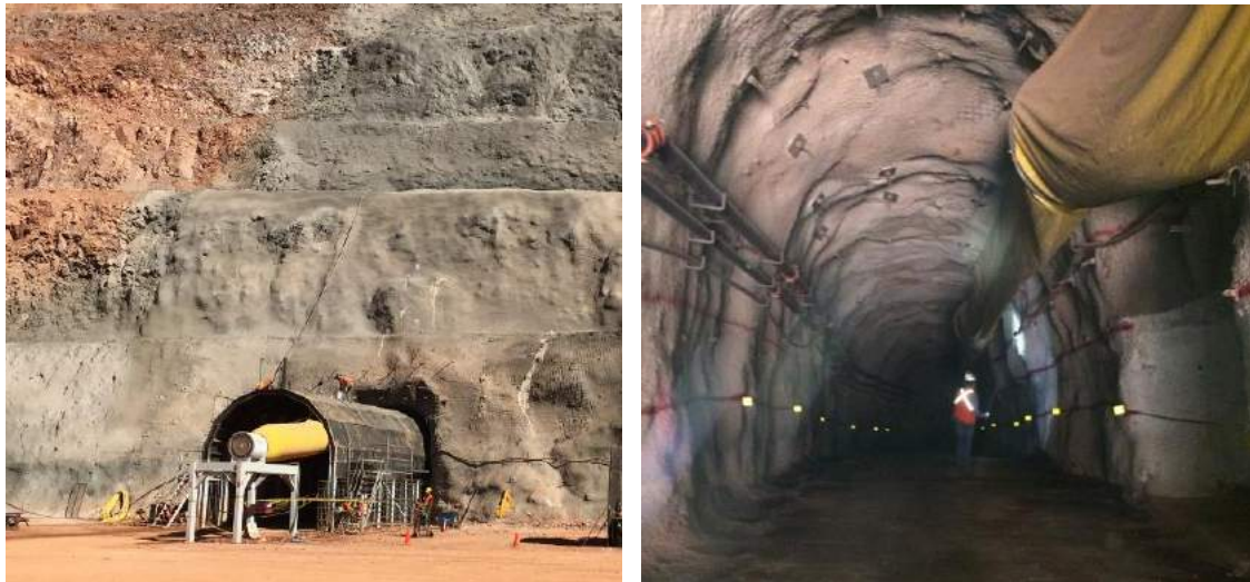
Figure 1a and b: Portal and Ramp for Development of Bermejil Underground
